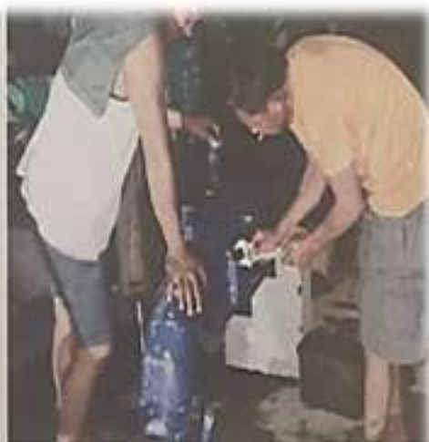
Re-installation of the submersible pump assembly well head
